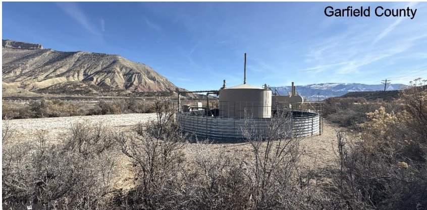
South West corner of location.
