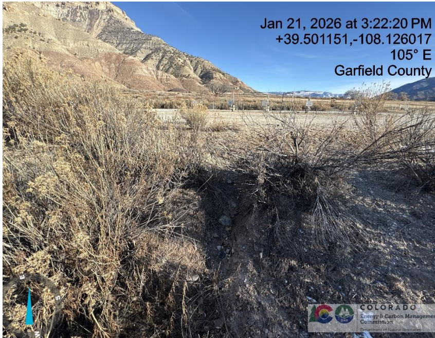
Photo # 3602 Berm needs maintenance/erosion & transport of sediment off location
