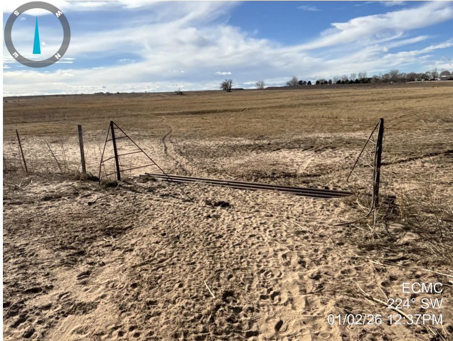
Photo 7. Photo taken of the access road to the well location, facing southwest. Photo illustrates that the access road remains unreclaimed with a cattle guard that is no longer in proper working condition.
