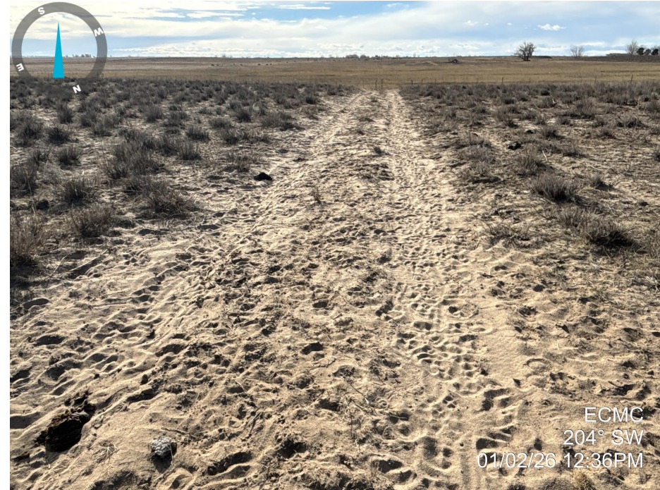
Photo 6. Photo taken of the access road to the well location, facing southwest. Photo illustrates that final reclamation activities do not appear to taken place along the access road as bare ground remains.
