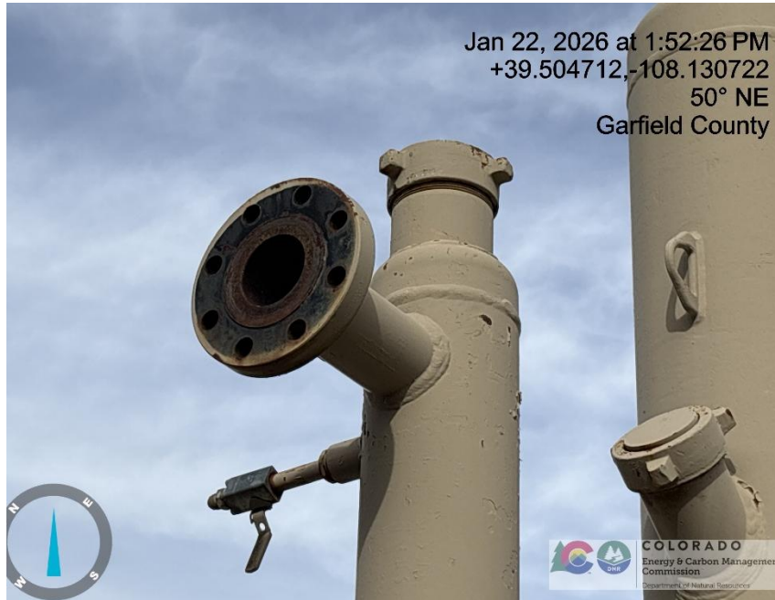
Photo # 4089 Flanged piping on separator unit open ended /wildlife hazard/available for entry by wildlife
