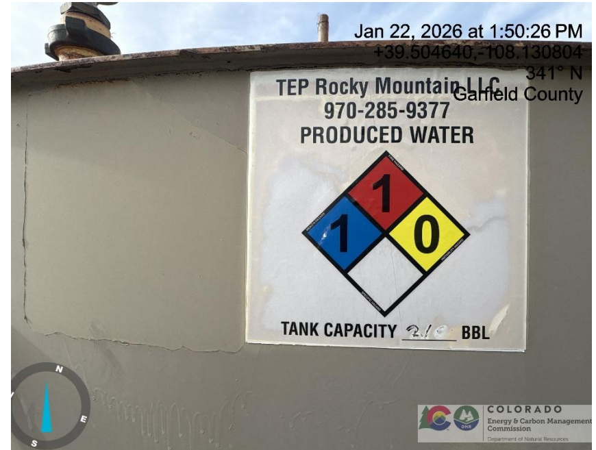
Photo # 4090 Capacity on tank label faded & becoming illegible
