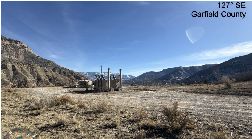
North West corner of location.
