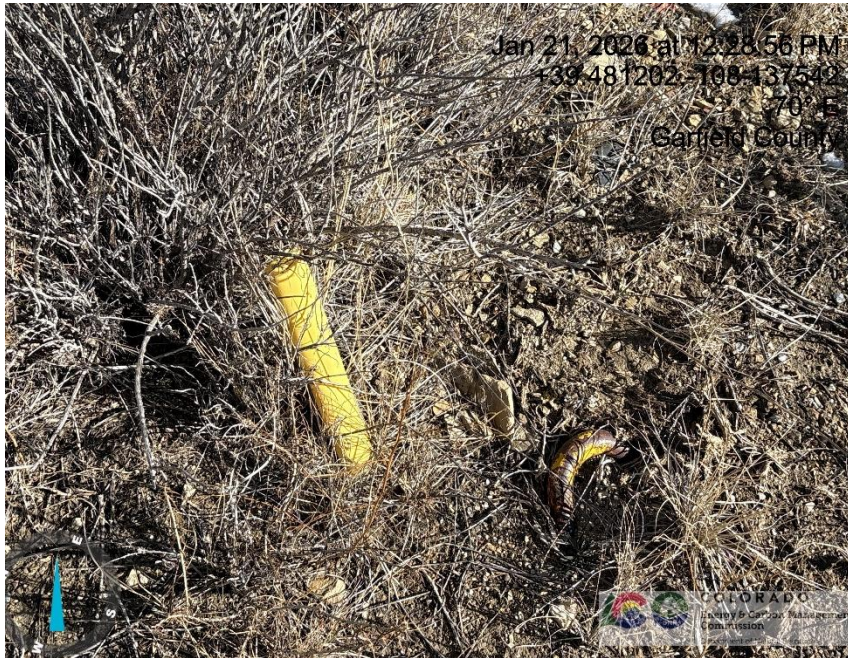
Photo # 3167 Improperly marked deadman
