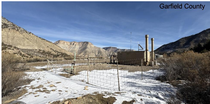
South West corner of location.
