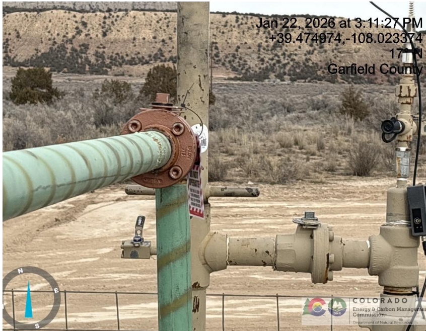
Photo # 4389 Observed valve on BH line going to ECD closed & tagged out
