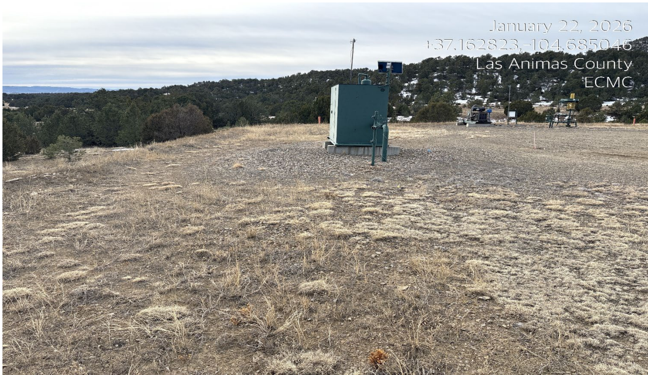
Photo 4. Facing south along the fill slope.
