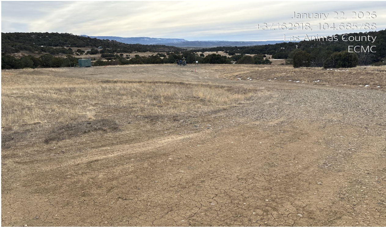
Photo 2. Facing southeast toward the wellsite.
