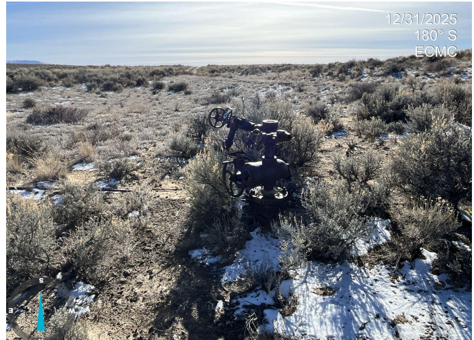
Photo 2. Photos 2-3 taken of the wellhead; equipment has not been removed.
