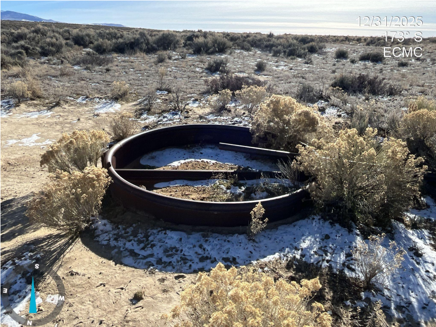
Photo 5. Photos 5-6 shows that pipe equipment remains on Location; it appears to have previously connected to the wellhead.
