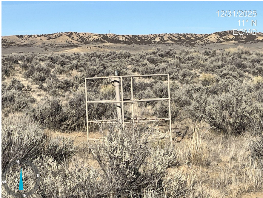
Photo 9. Photo taken of risers near the access road, which have not been removed.
