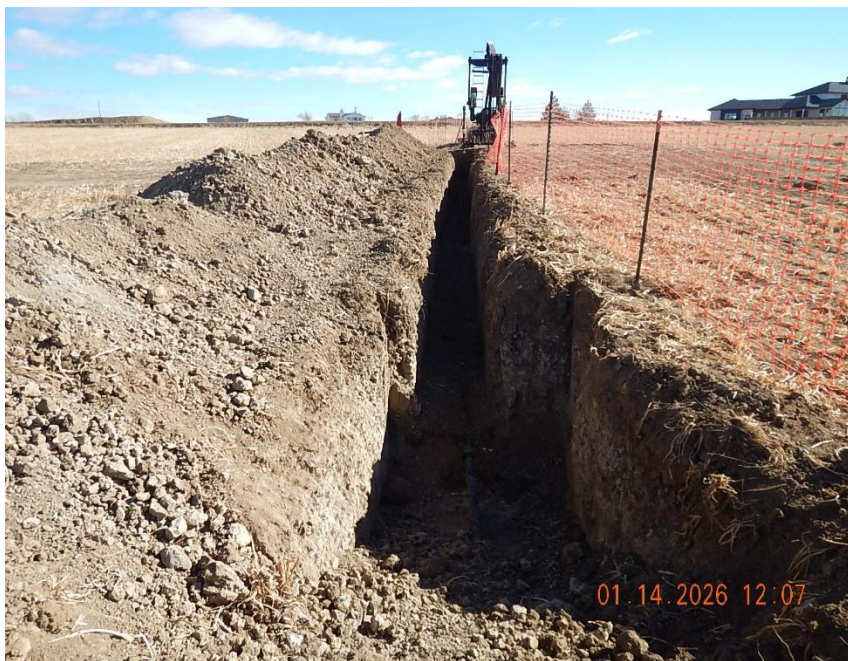
Flowline trench western endpoint @ 40.06798, -104.945571 View looking east
