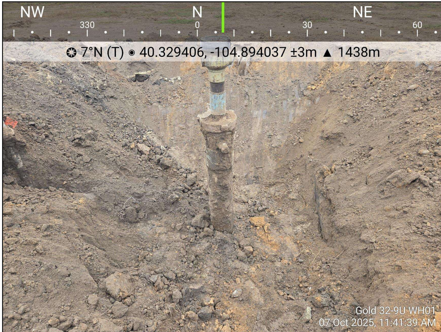
Photo 2: View of excavation extent, facing north
