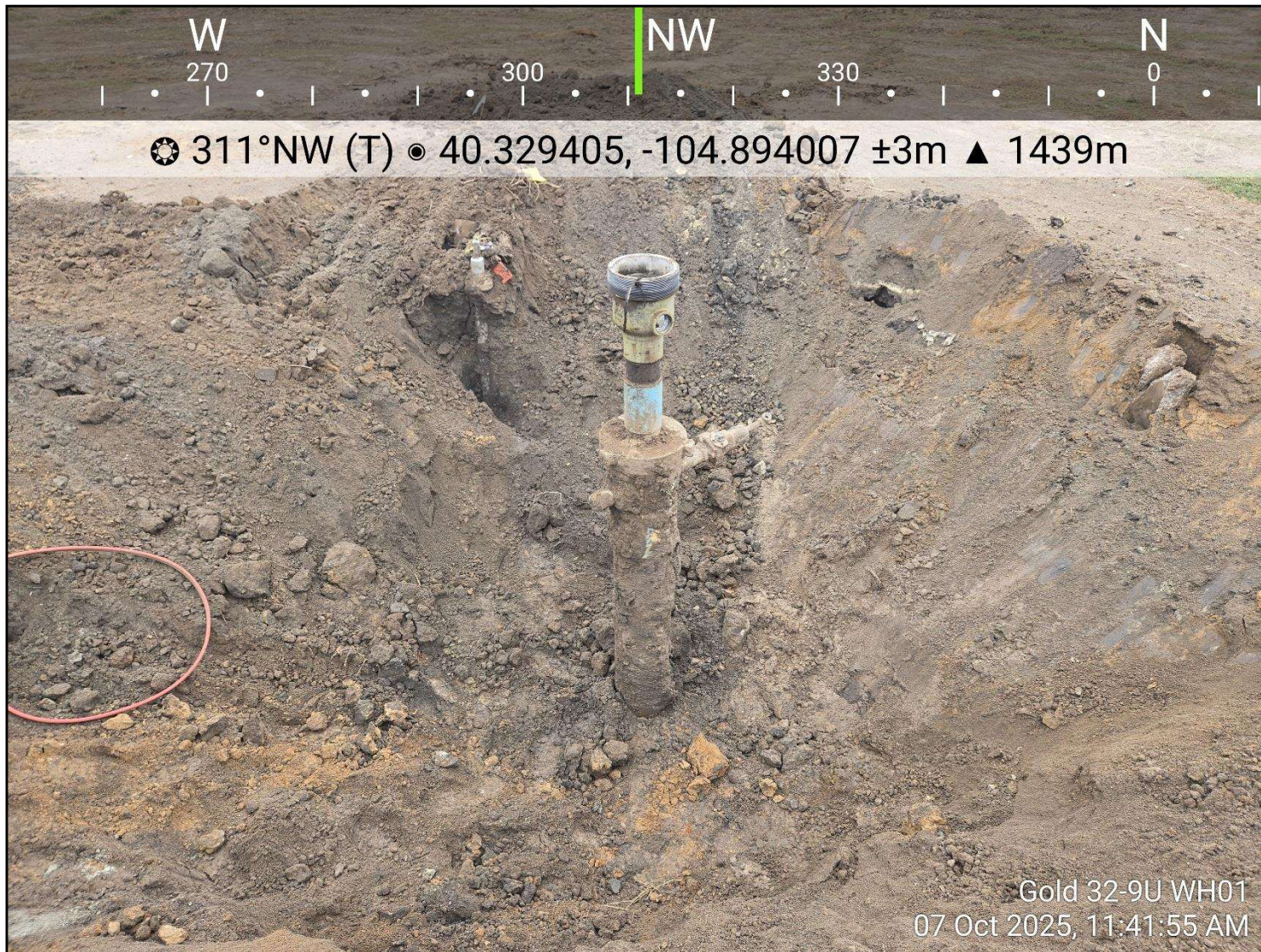
Photo 5: View of excavation extent, facing northwest
