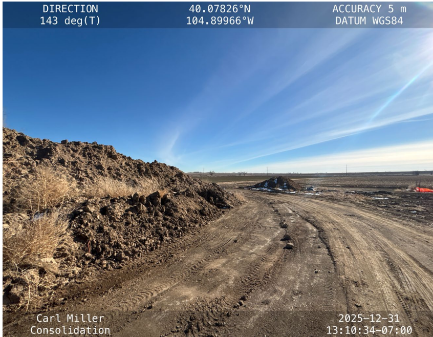
Stockpile no liner of BMPs
