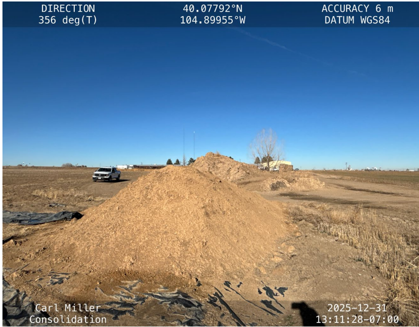
Stockpile with liner torn
