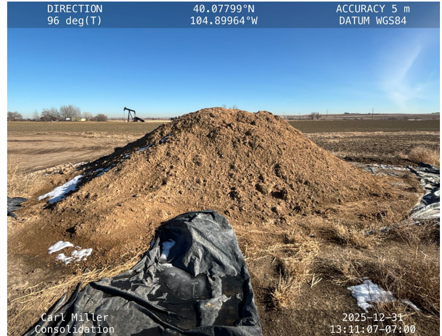
Stockpile with liner torn
