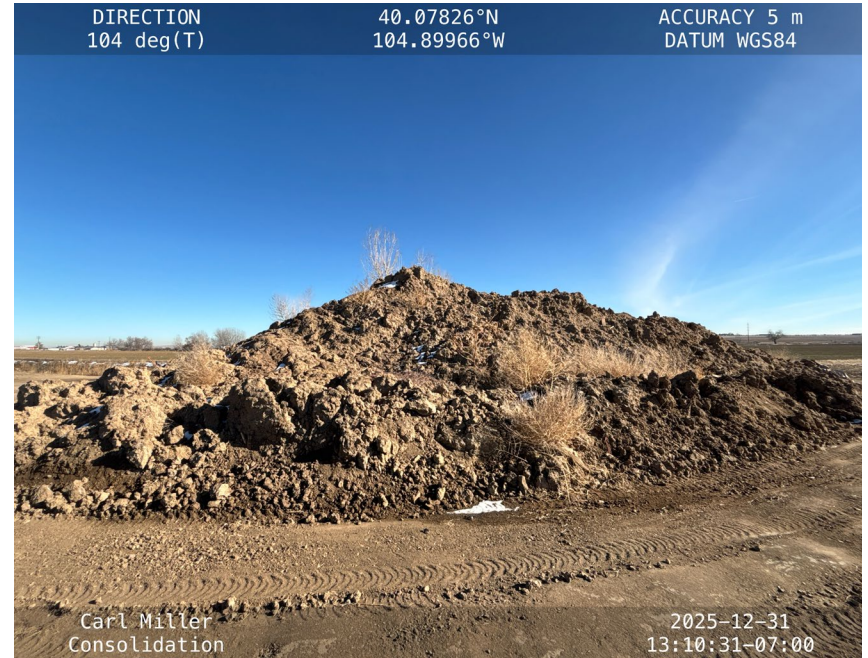
Stockpile no liner of BMPs
