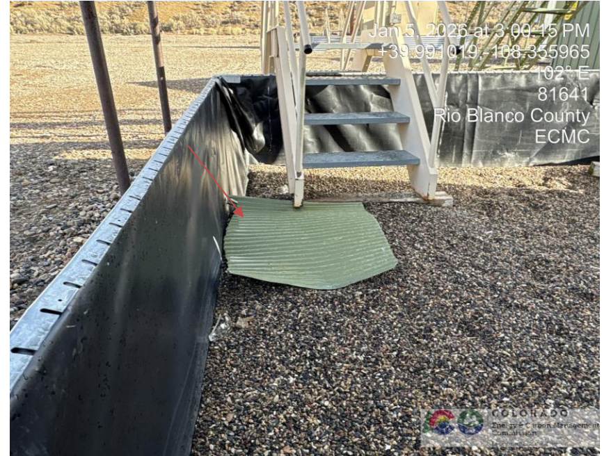
Photo # 0555 Debris on location
