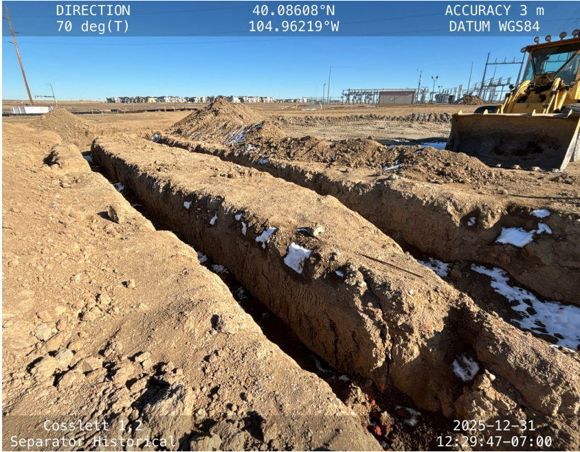
Excavation with inadequate fencing
