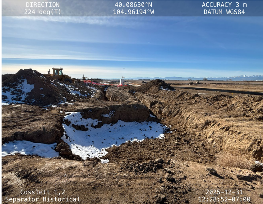
Excavation with inadequate fencing
