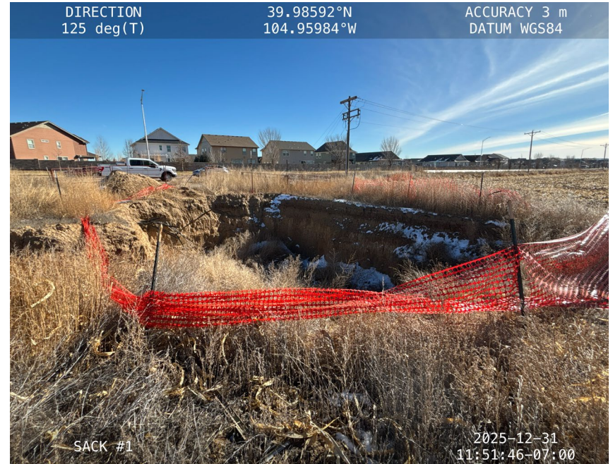
Excavation with fallen fencing
