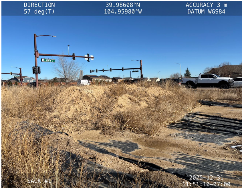
Stockpile with weeds and torn liner
