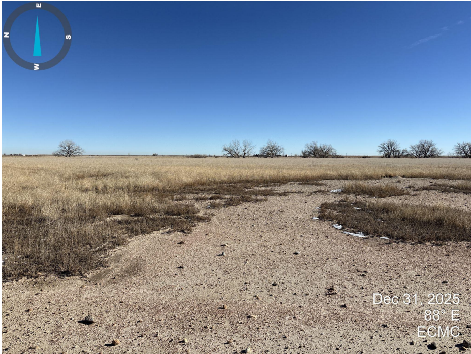
Photo 5. Looking east from the center of the well turnaround area. See photo 4 comments.
