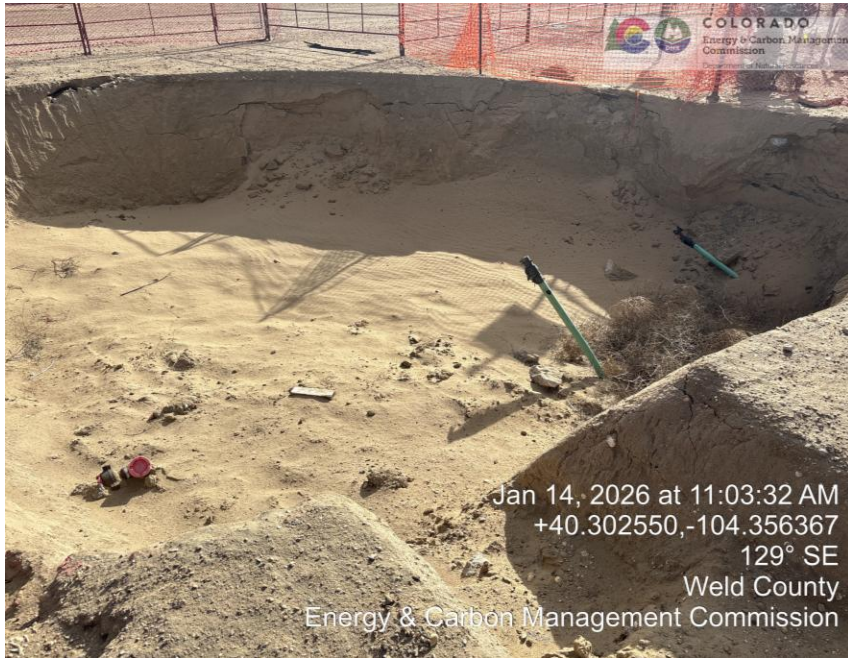
Photo 1 well head remediation area
