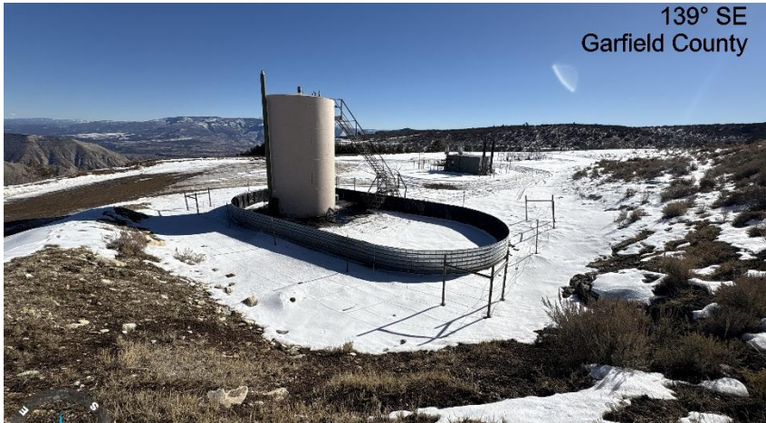
North West corner of location.
