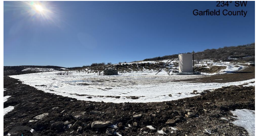
North East corner of location.
