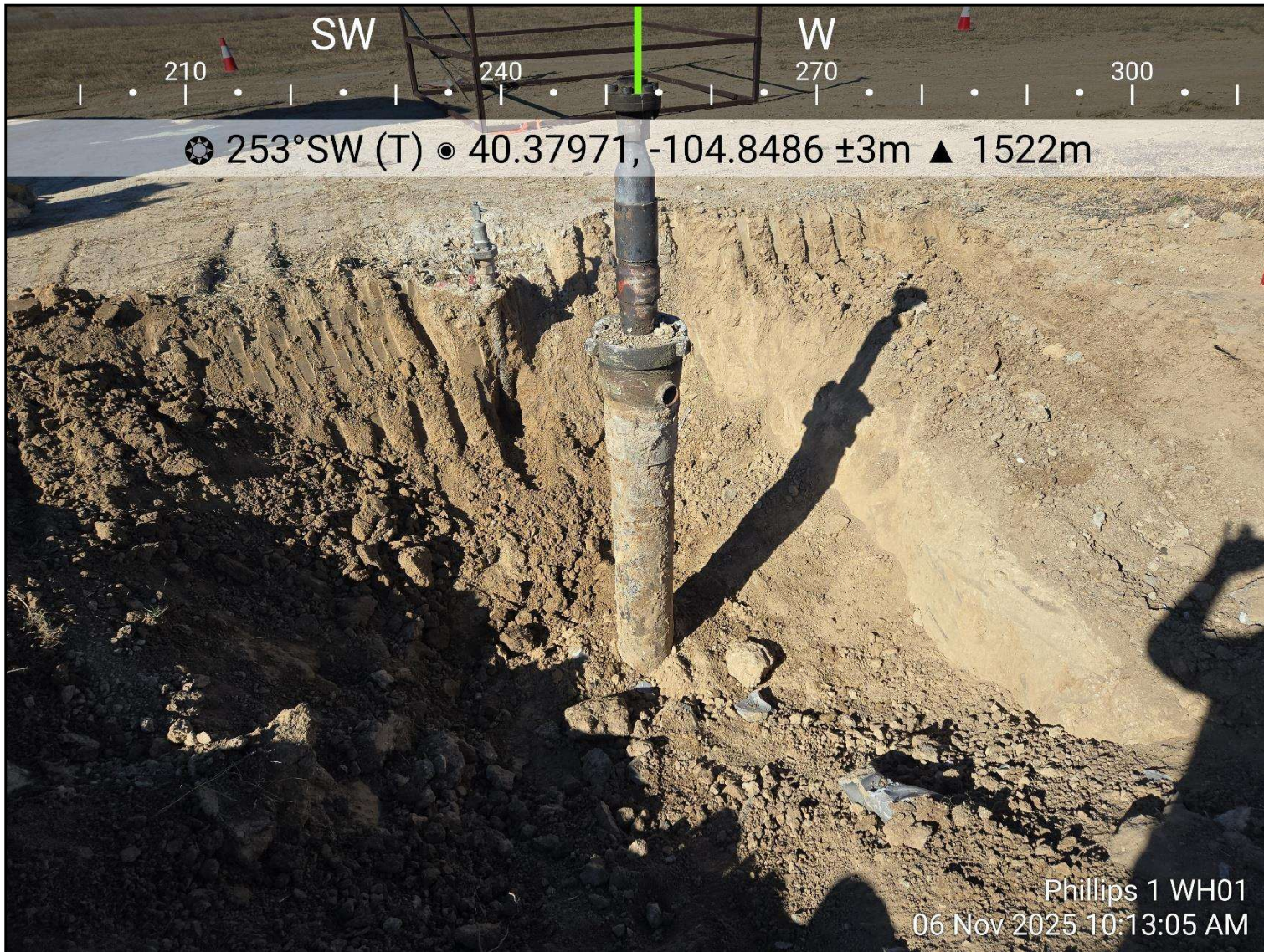
Photo 4: View of wellhead excavation, facing west-southwest
