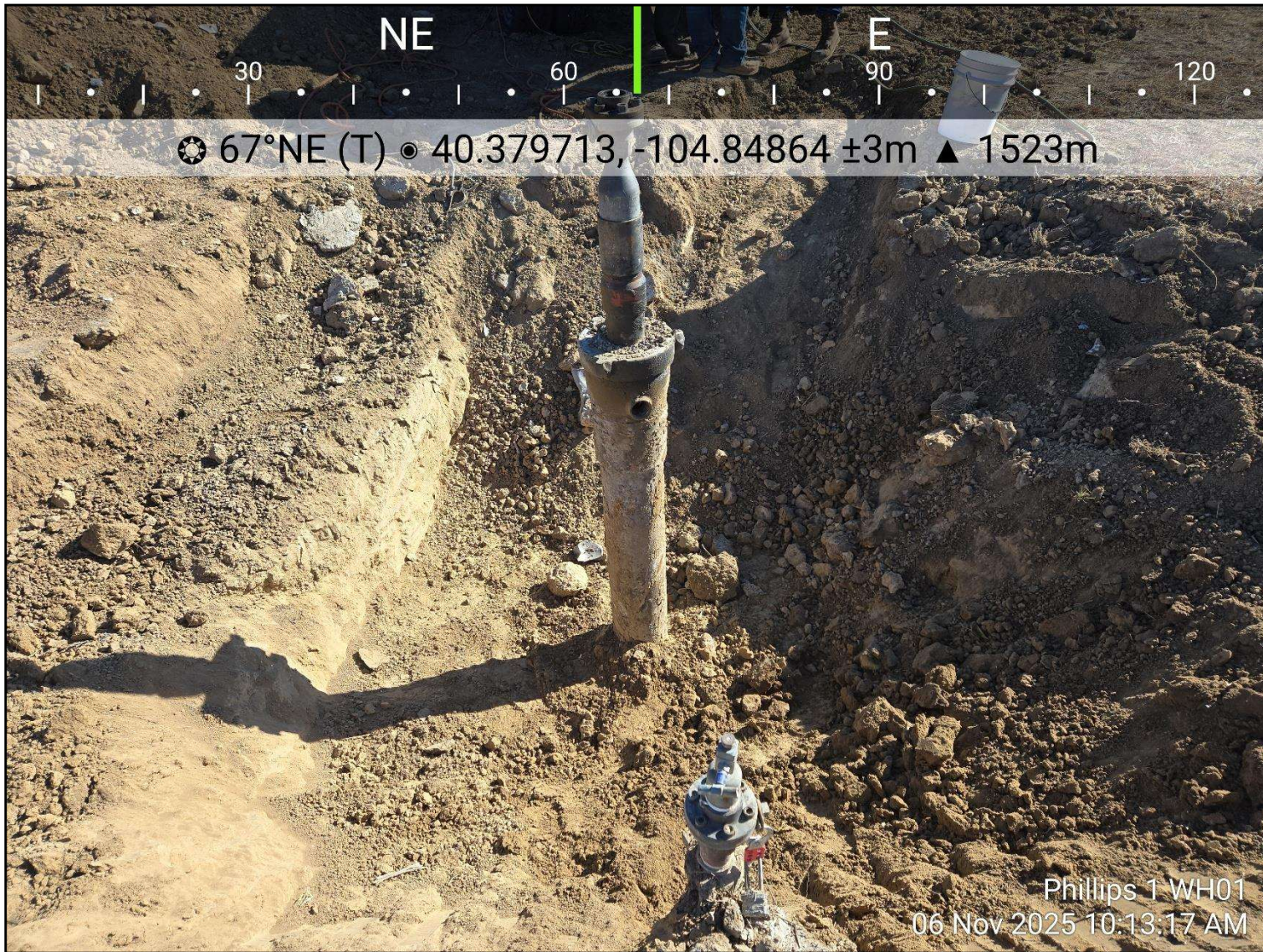
Photo 2: View of wellhead excavation, facing east-northeast
