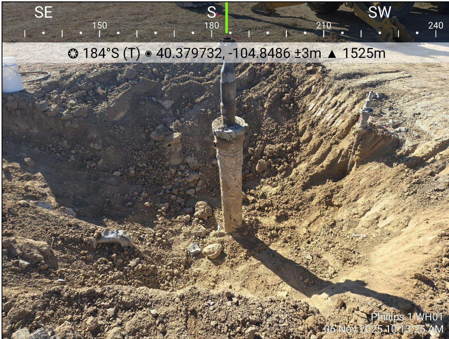
Photo 1: View of wellhead excavation, facing south
