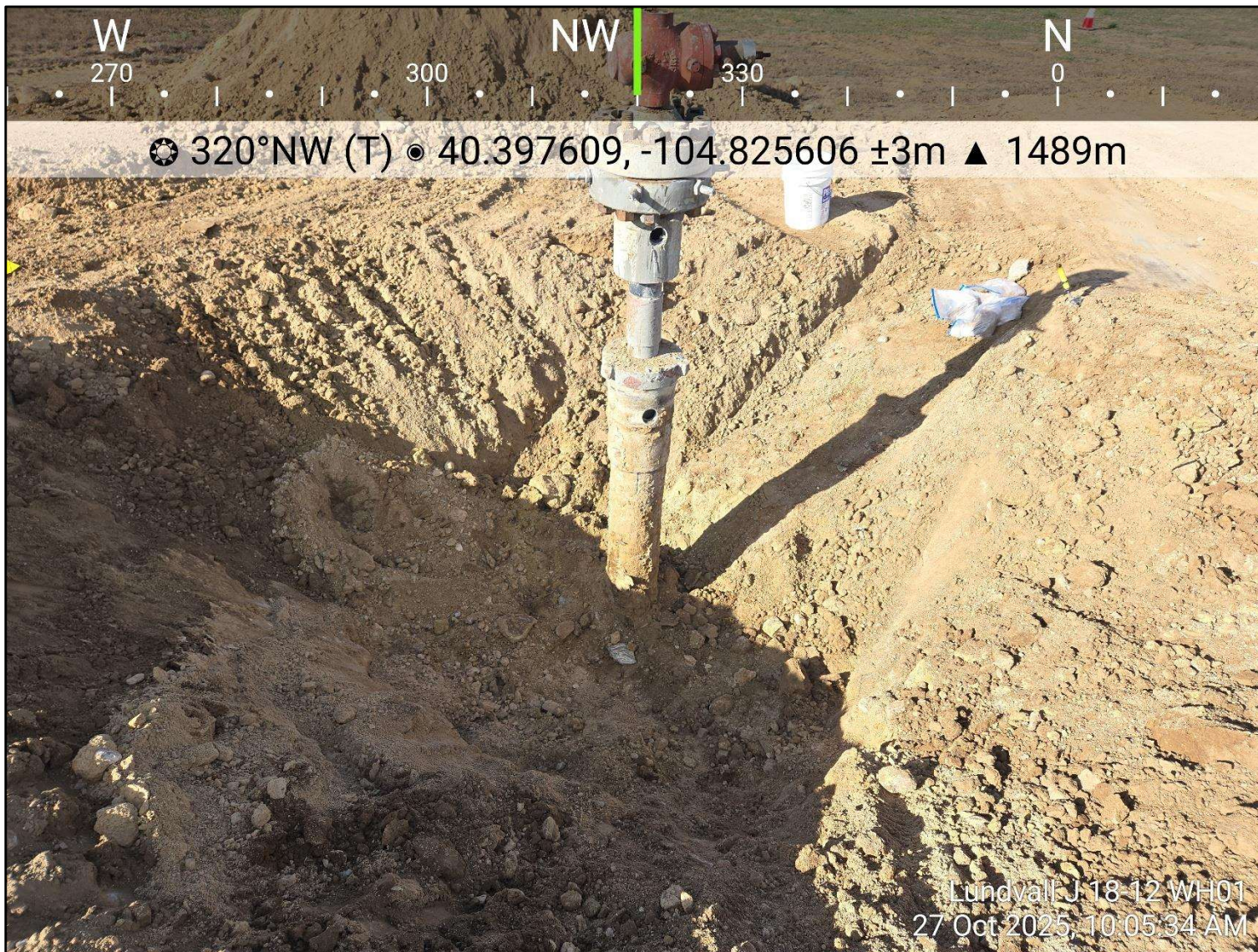
Photo 2: View of wellhead excavation, facing northwest
