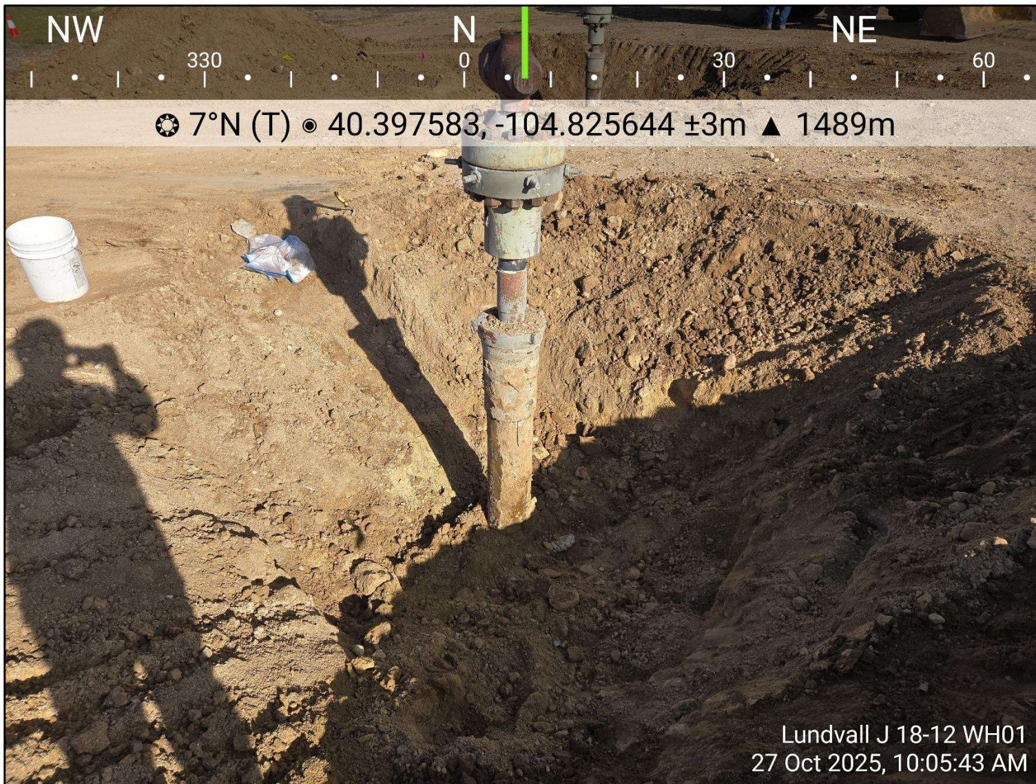
Photo 1: View of wellhead excavation, facing north
