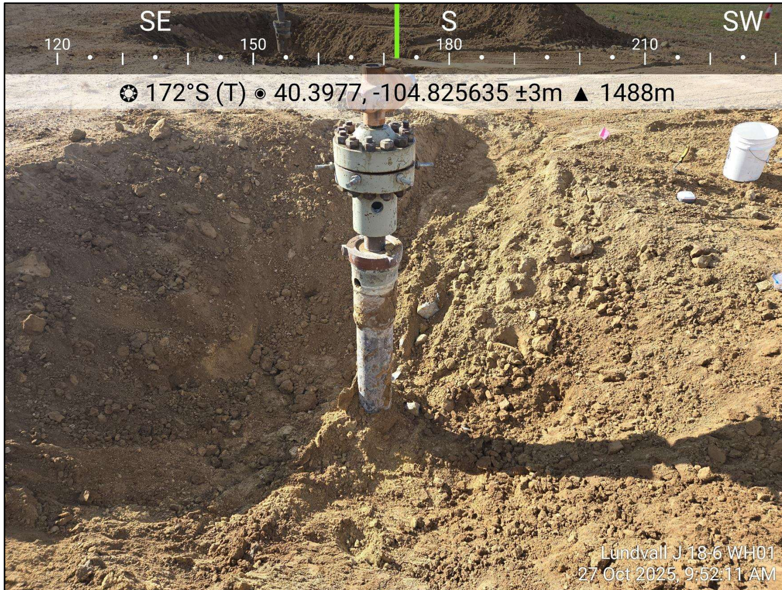
Photo 3: View of wellhead excavation, facing south
