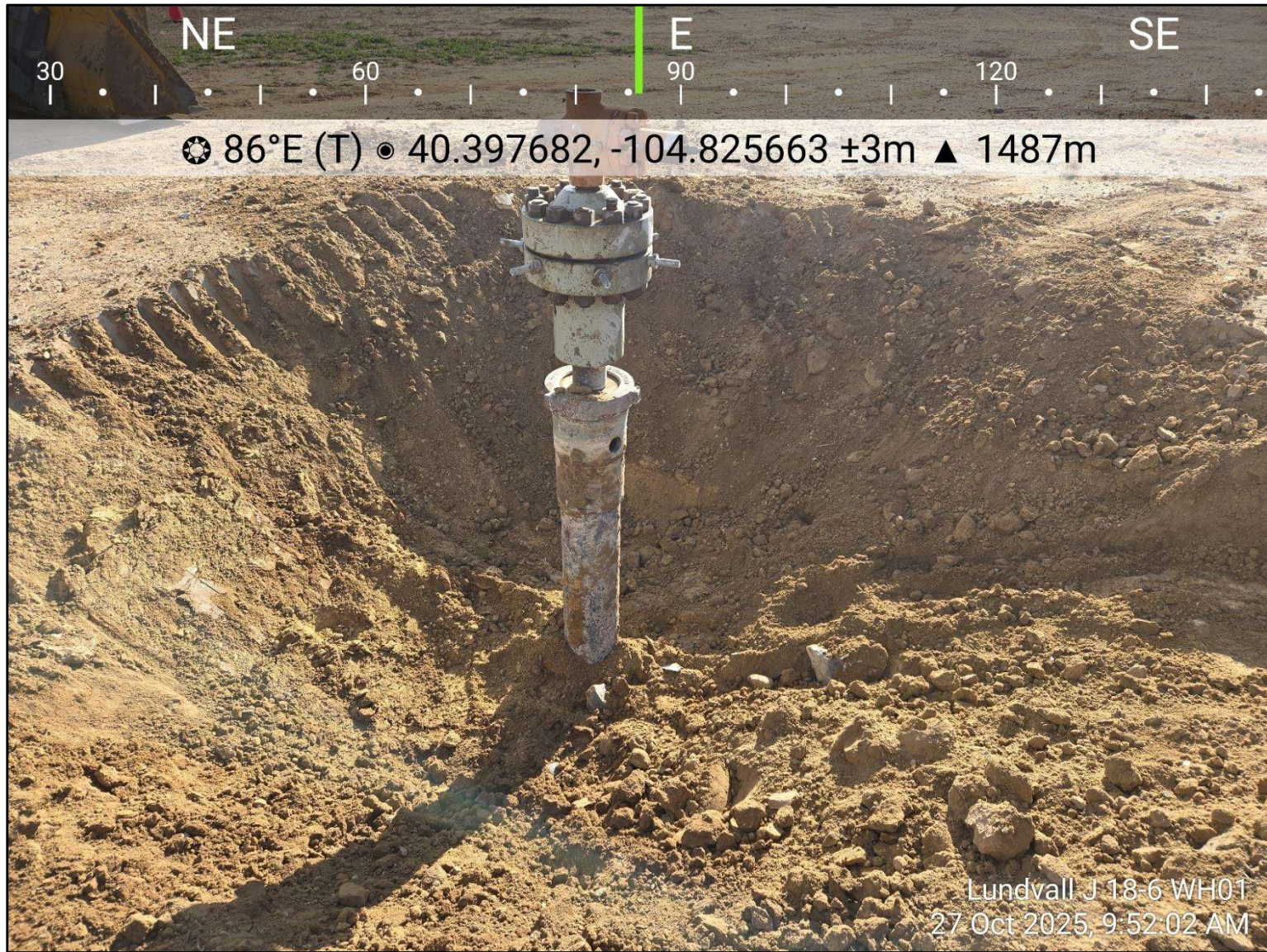
Photo 4: View of wellhead excavation, facing east
