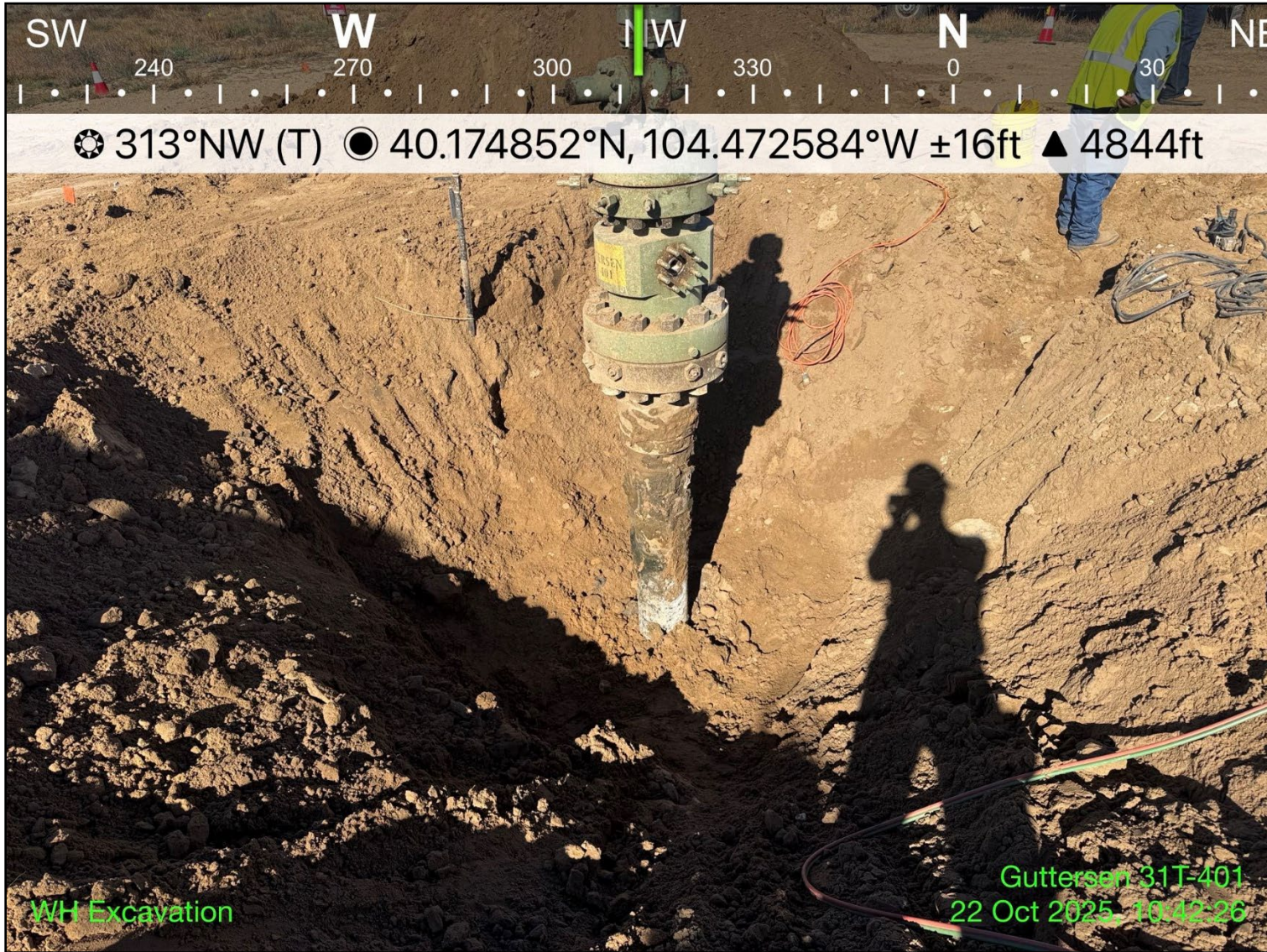
Photo 4: View of wellhead excavation extent, facing northwest
