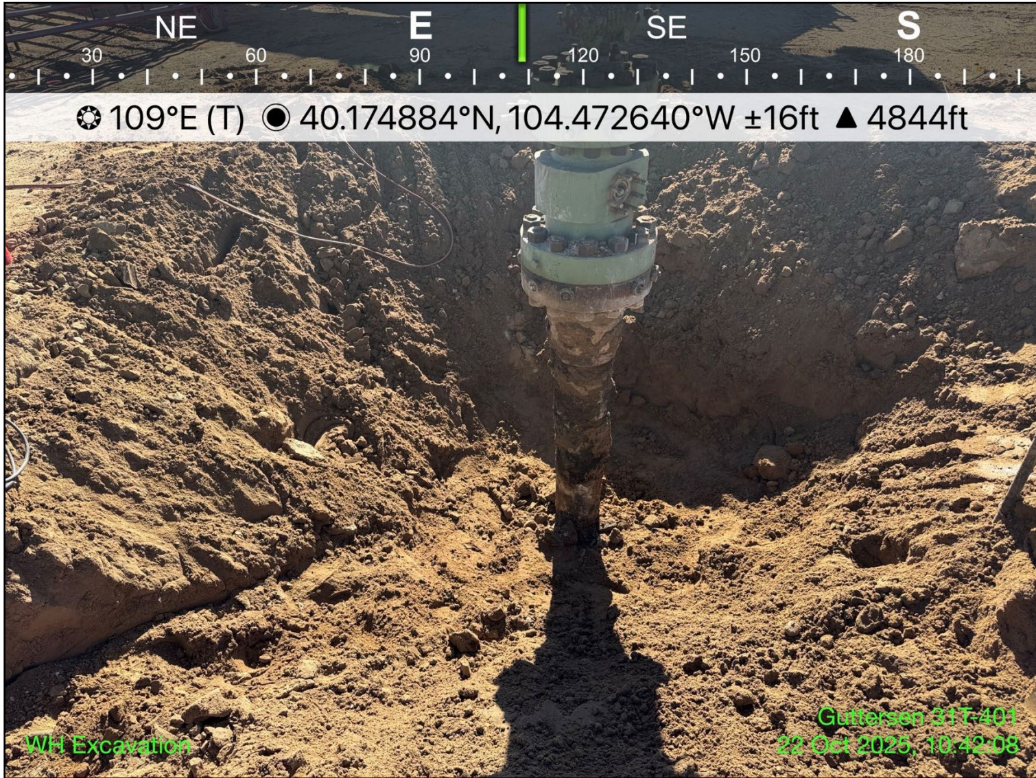
Photo 3: View of wellhead excavation extent, facing east-southeast
