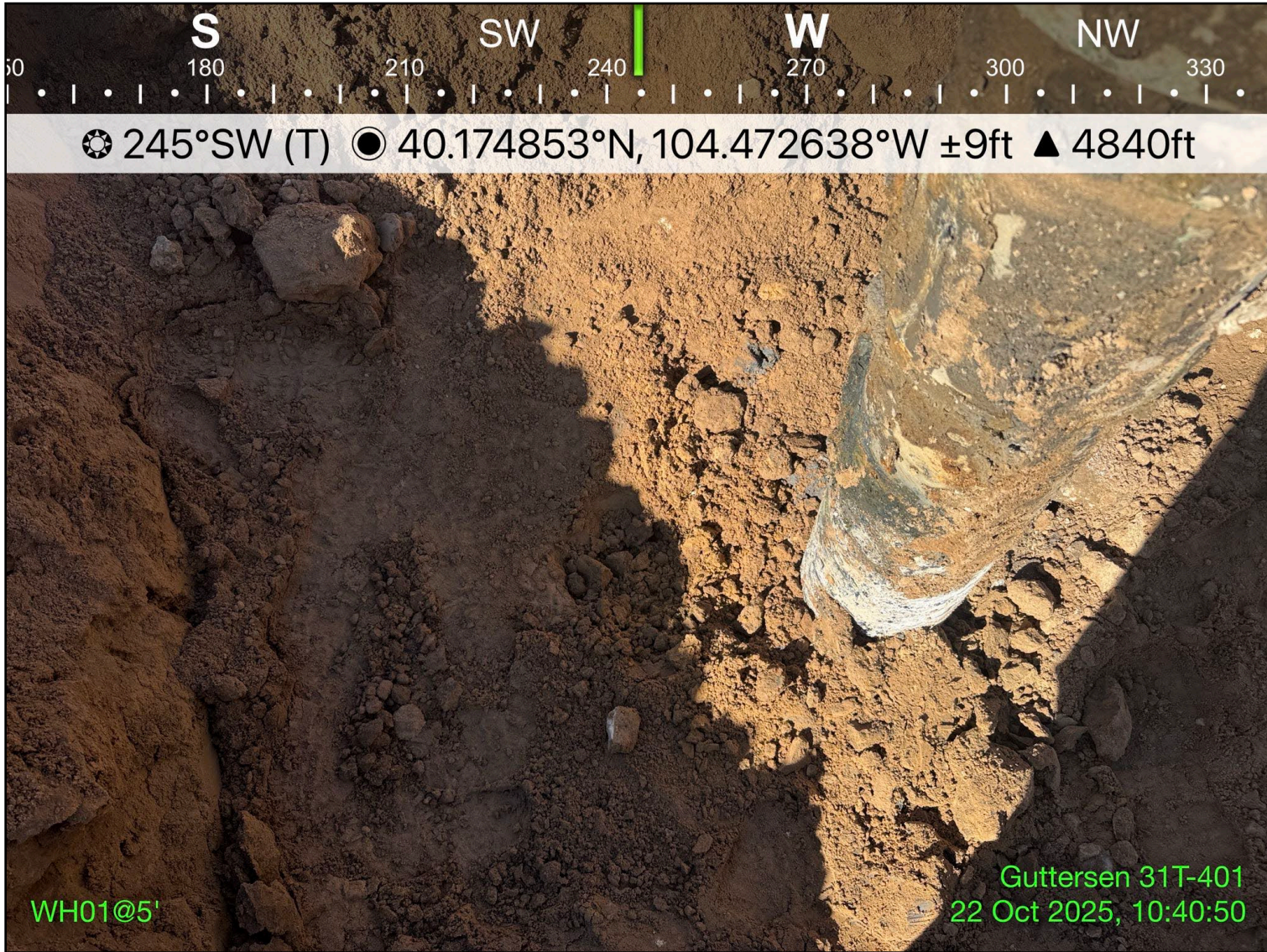
Photo 1: View of wellhead excavation extent, facing west-southwest
