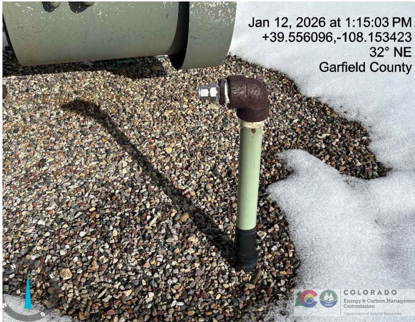
Photo # 99 Unused flowline lacks lockout tagout (OOSLAT) Line is located in secondary containment near tank heater
