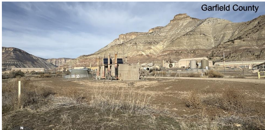
South West corner of location.
