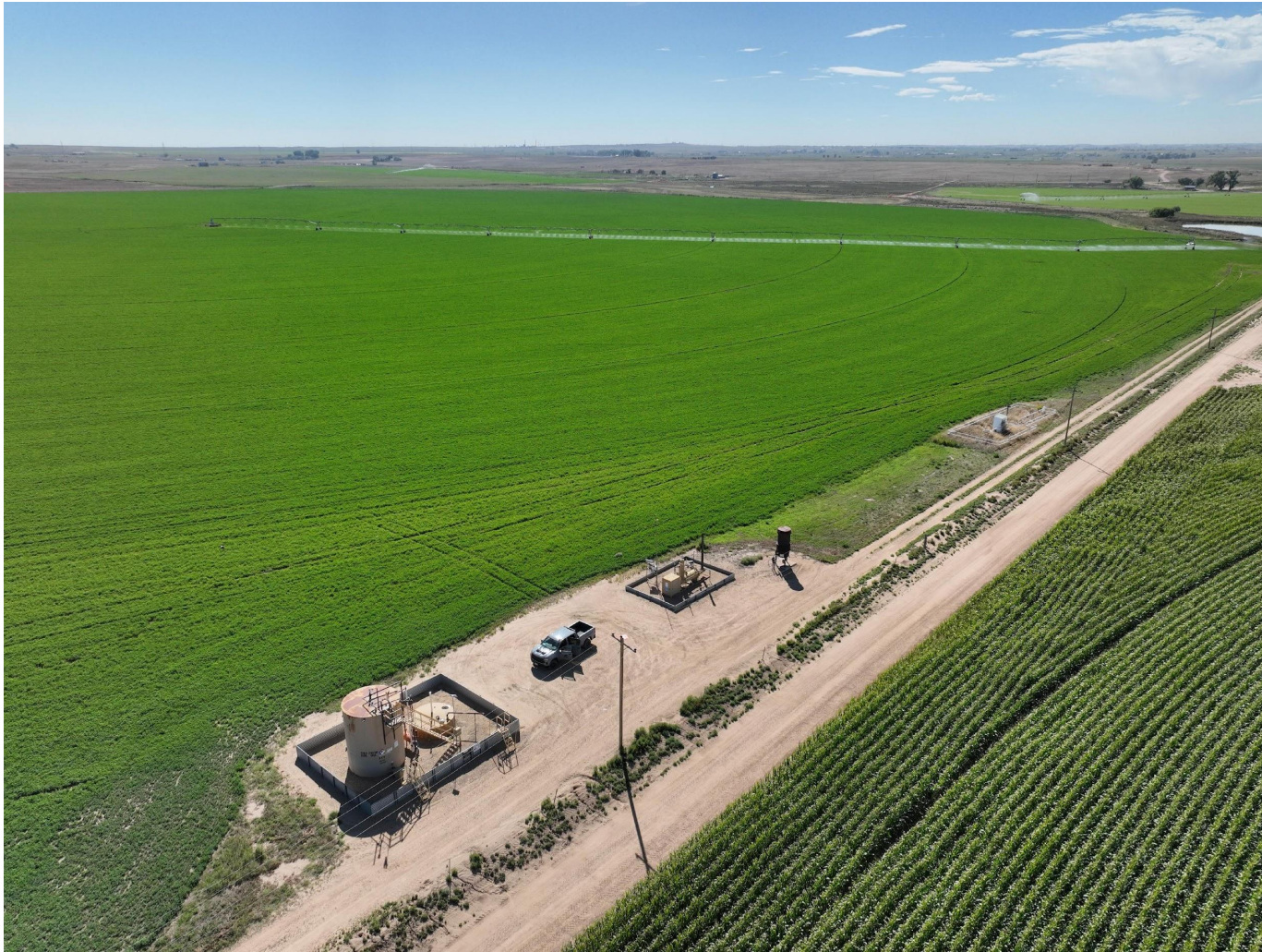
Photo 10. Drone imagery of active tank battery.
