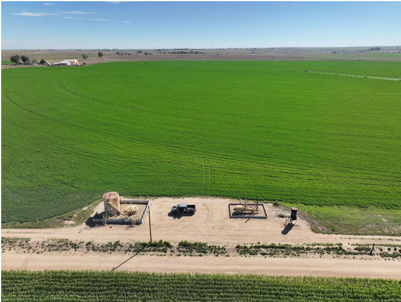
Photo 8. Drone imagery of the active tank battery,.
