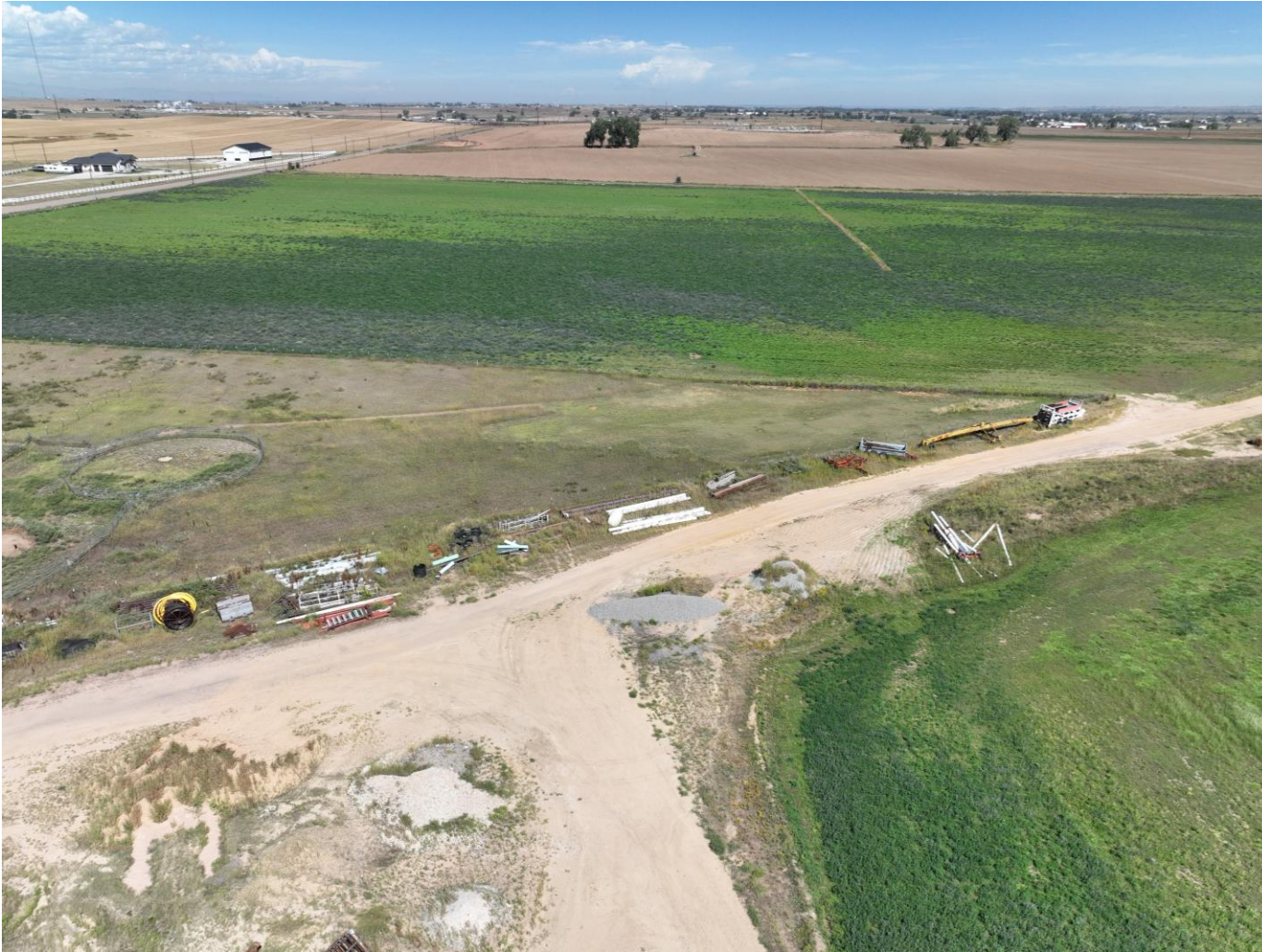
Photo 8. Drone aerial imagery taken south of the tank battery location, facing north (displaying the TB).
