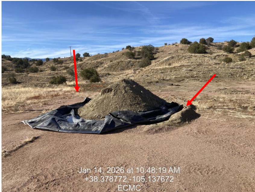
Photo 5 – Impacted spoil pile in containment
