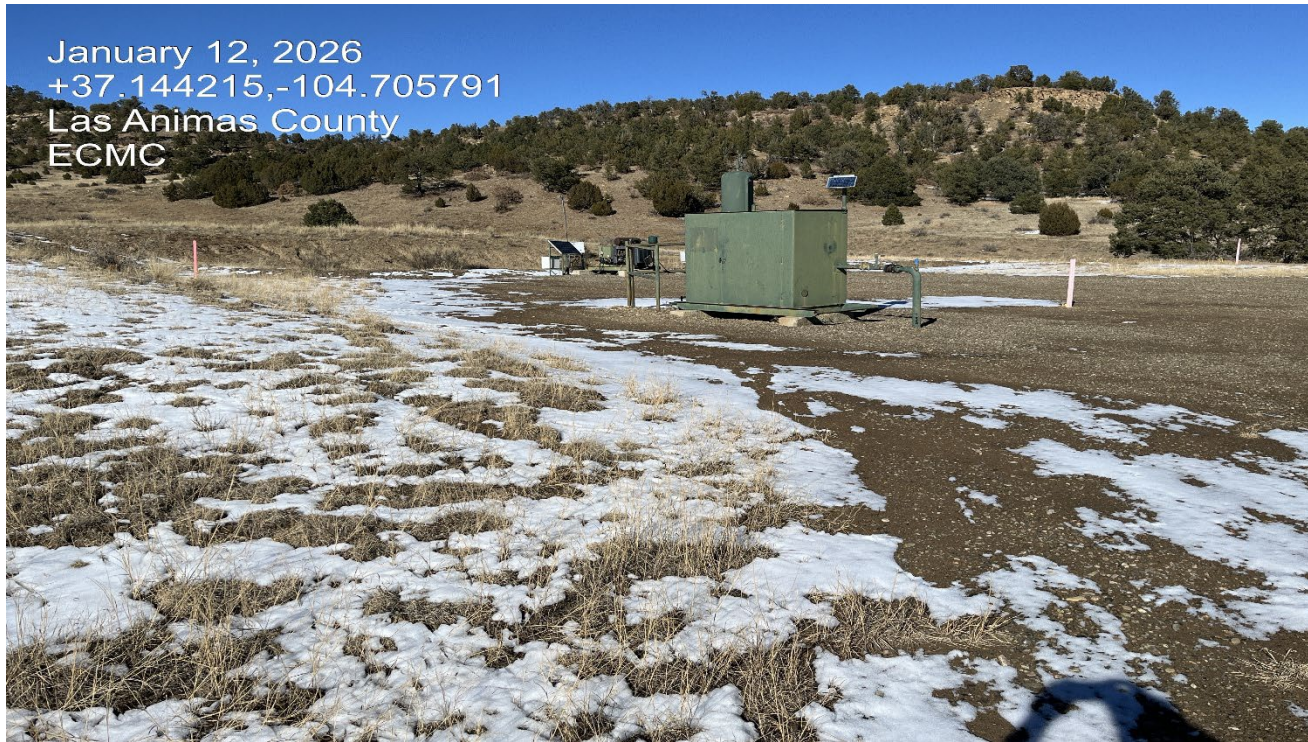
Photo 1. Facing northeast toward the wellsite.
