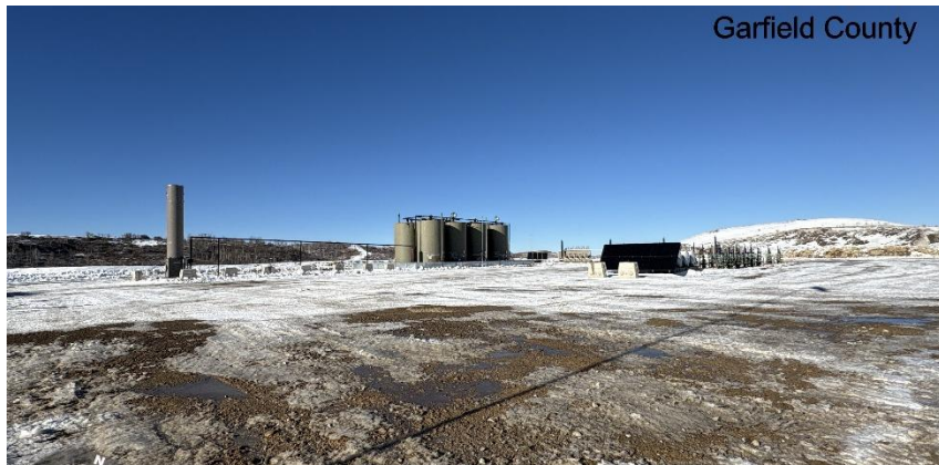
South West corner of location.
