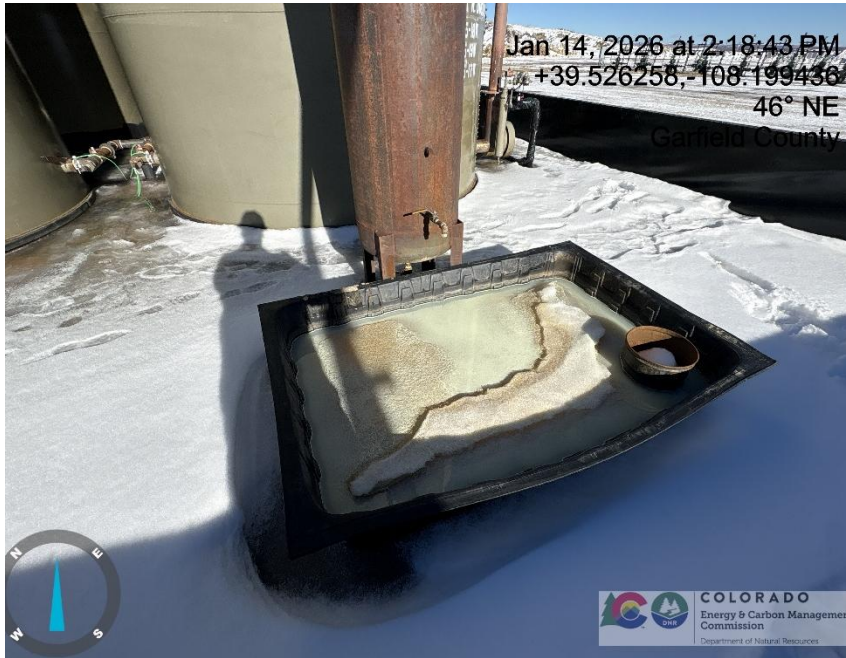
Photo # 1293 Plastic containment containing unknown fluid lacks wildlife protection/wildlife hazard
