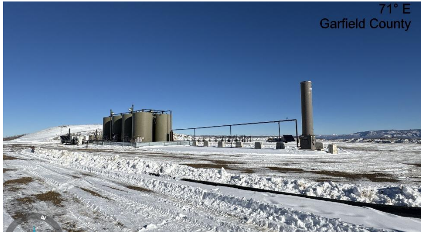
North West corner of location.
