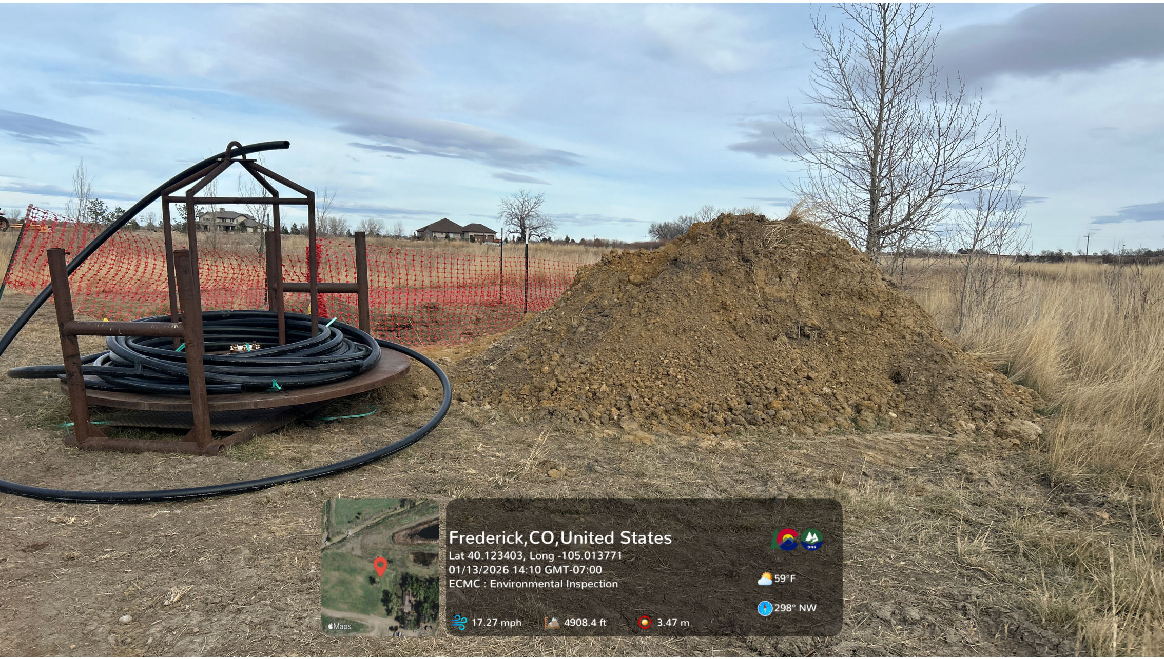
Looking at an unmarked, unlined soil stockpile with no stormwater BMPs which remains on location. Areas of gray staining are visible within the stockpile.
