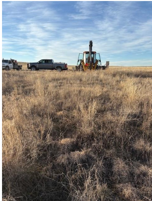
Photo 5. Middle of location facing W.
