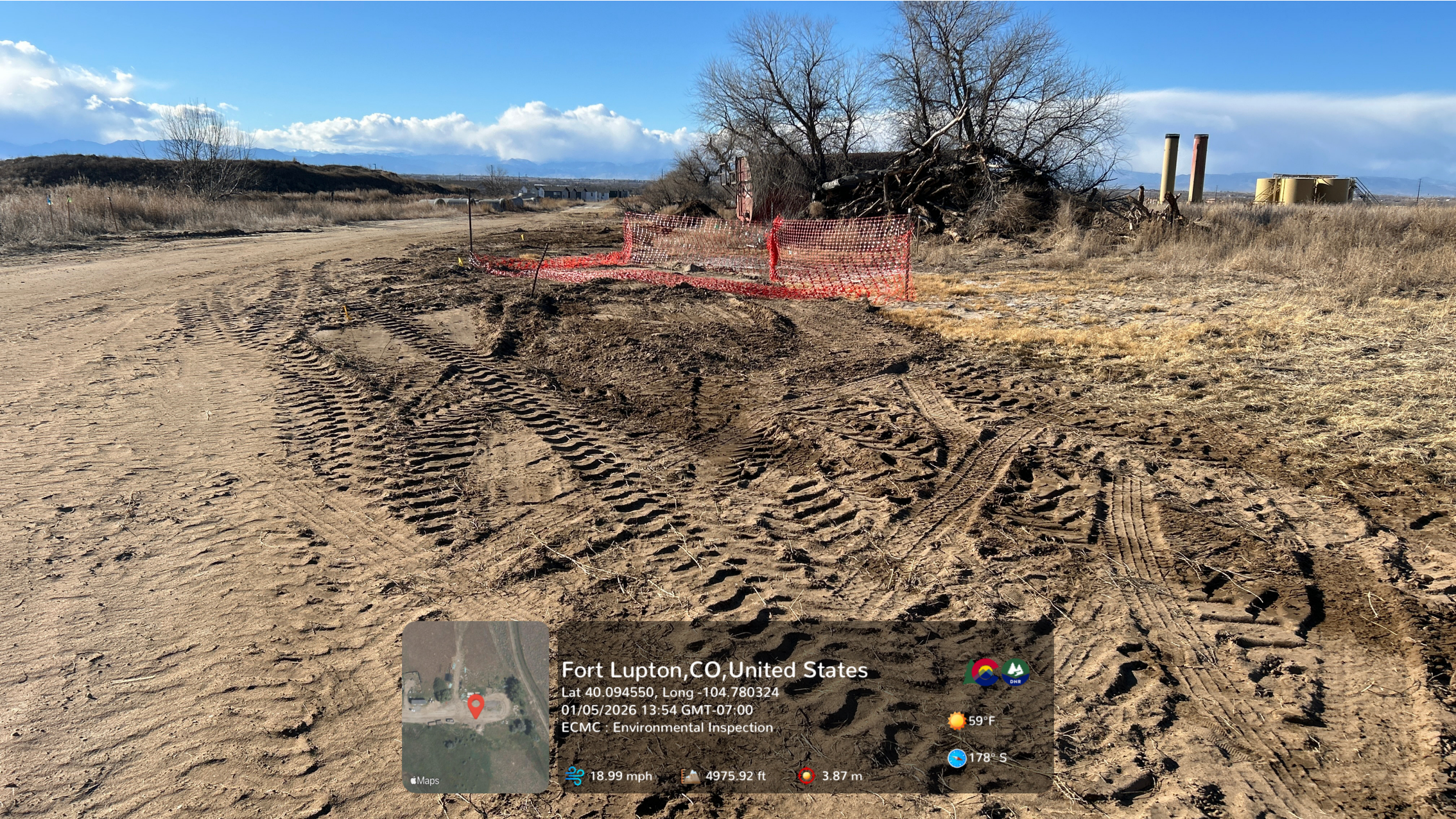
Looking along spill location, where Operator reports the fluid flowed after daylighting.
