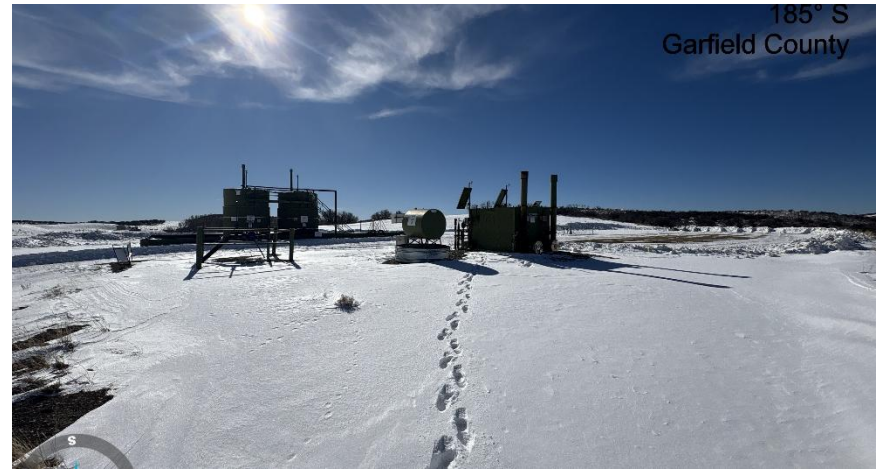
North East corner of location.
