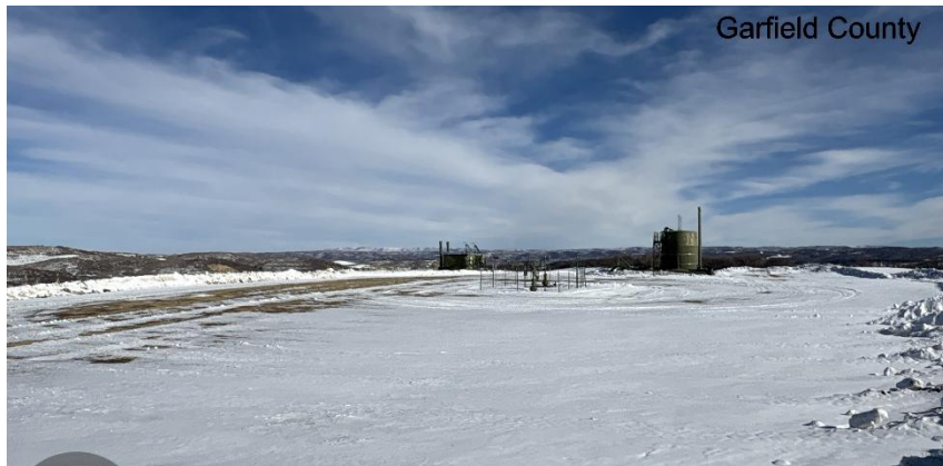
South West corner of location.
