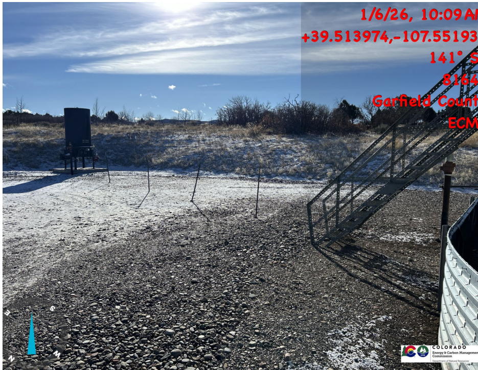
Main line from tanks to ECD disconnected and locked out
