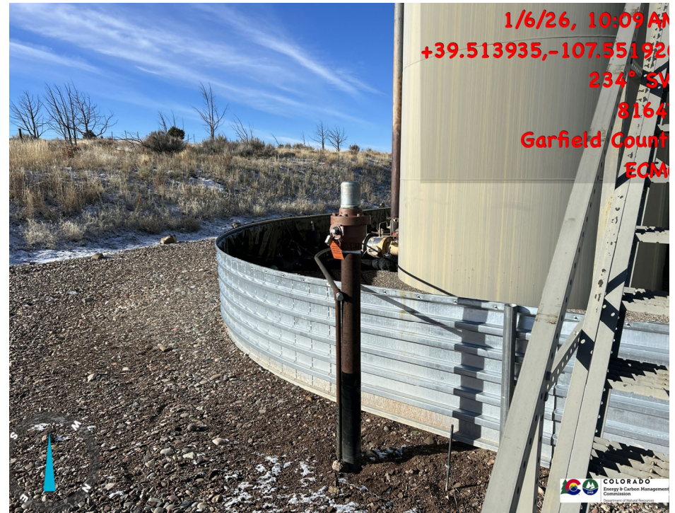
Main line from tanks to ECD disconnected and locked out
