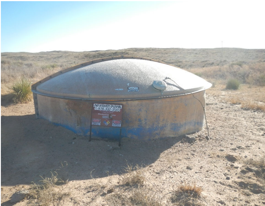
5. View of produced water tank at remote gathering location.
