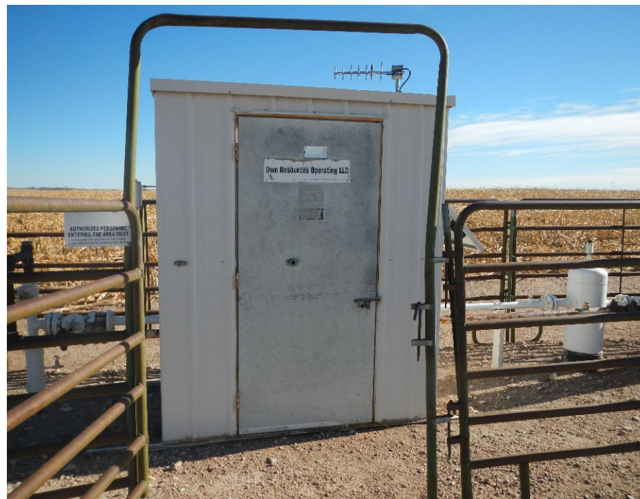
6. View of Gas Meter Run Shed.
