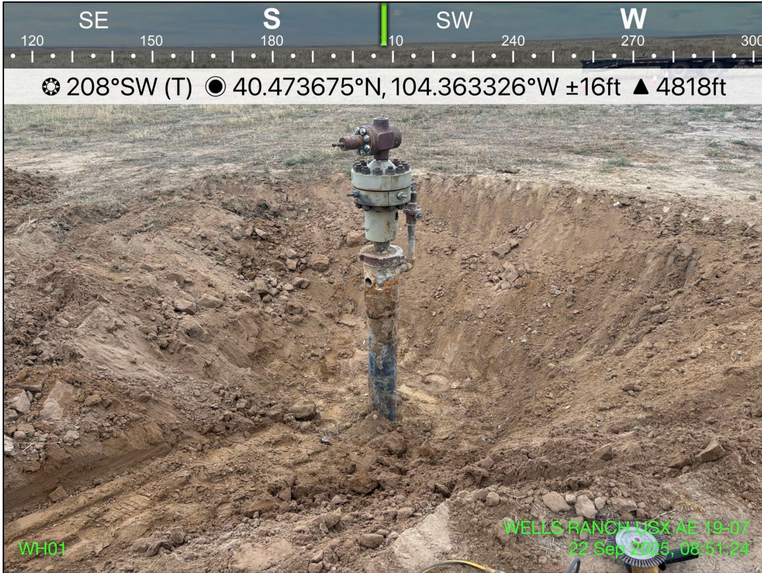
Photo 4: View of wellhead excavation area, facing south-southwest
