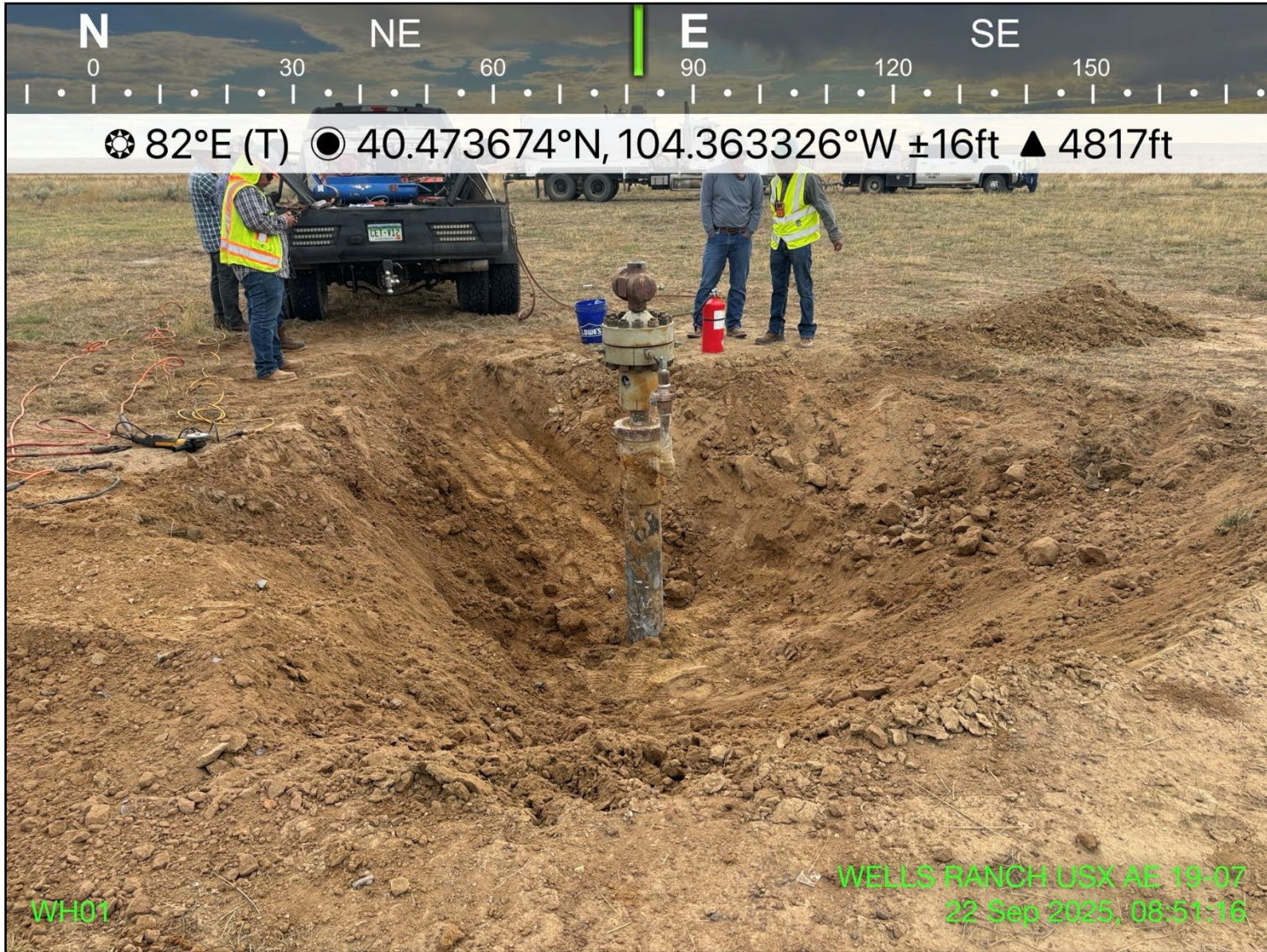
Photo 3: View of wellhead excavation area, facing east
