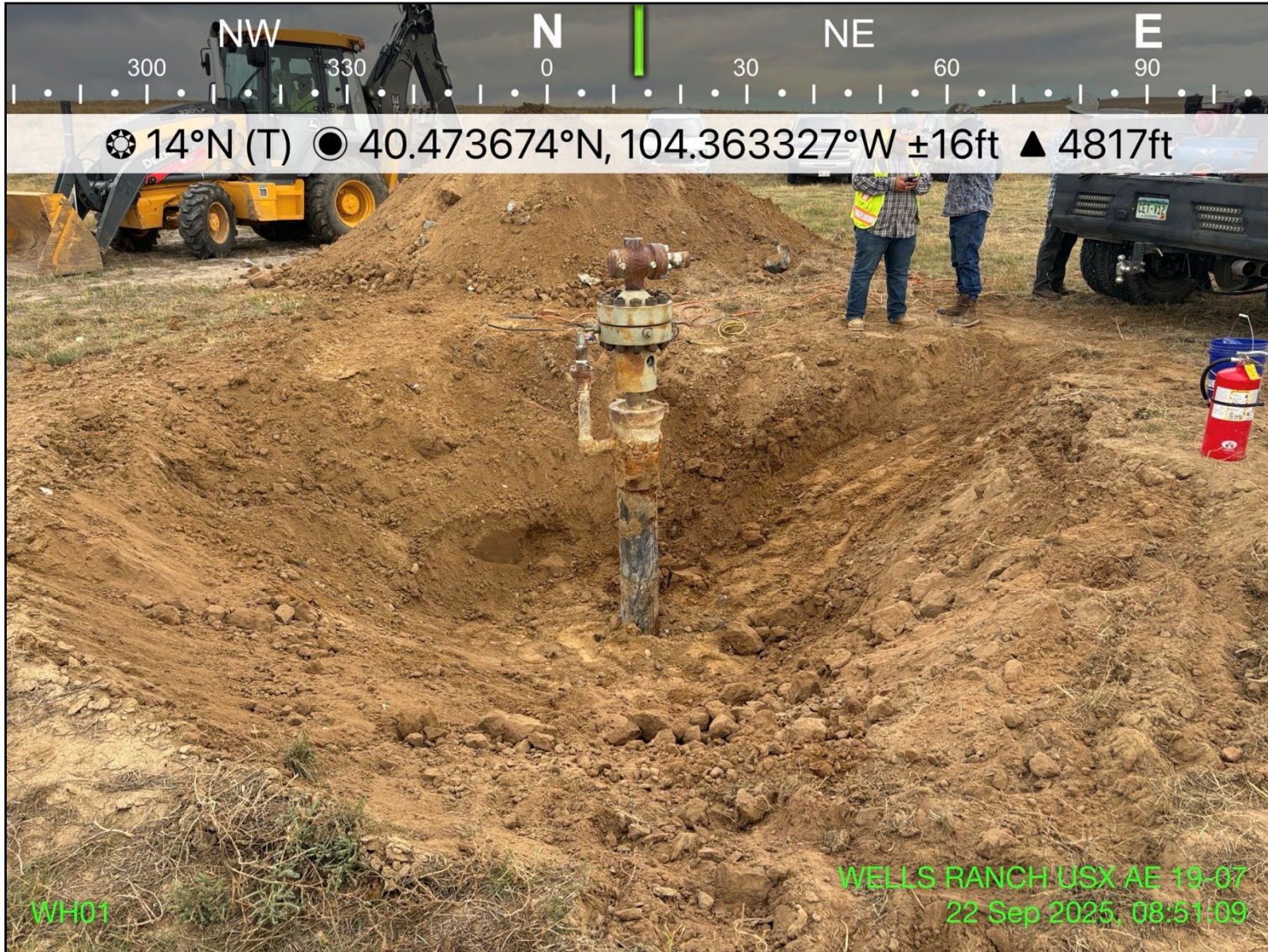
Photo 2: View of wellhead excavation area, facing north
