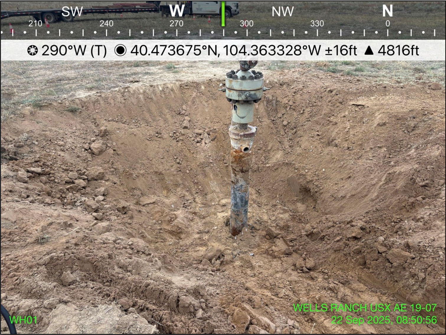
Photo 1: View of wellhead excavation area, facing west-northwest
