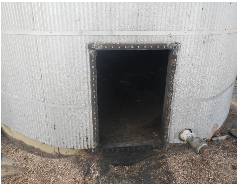
7. Production tank entry hatch removed. Note hydrocarbons on ground outside of entry. No caution or warning signs in place.
