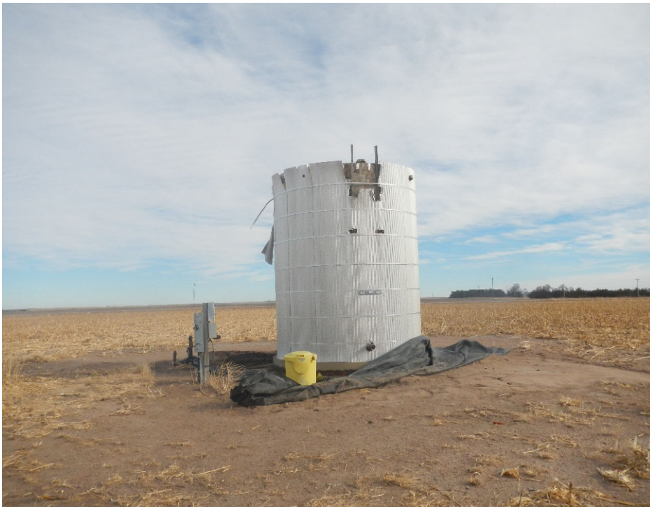
5. View of production tank.
