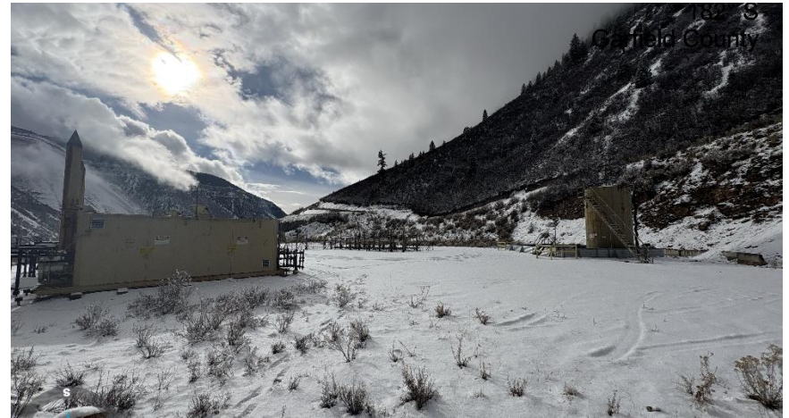
North East corner of location.
