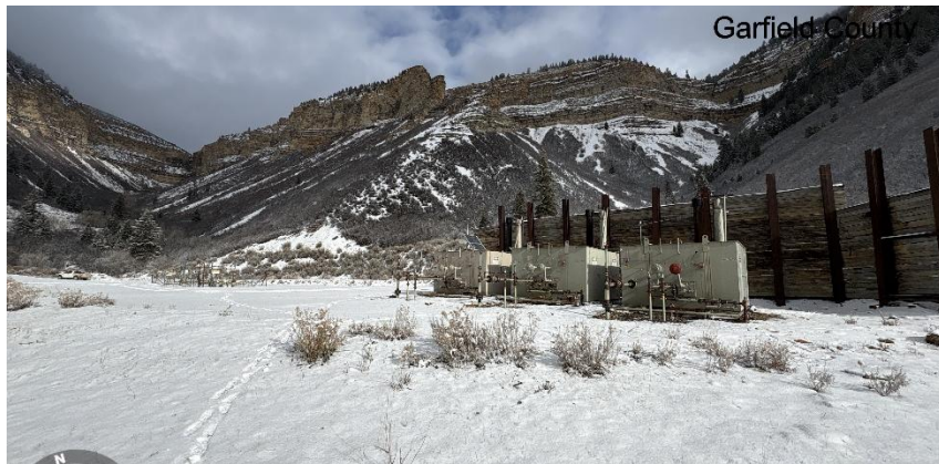
South West corner of location.
