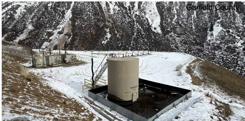
South West corner of location.
