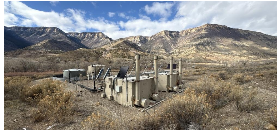
South East corner of location.
