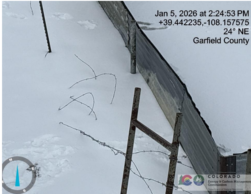
Photo # 8112 Barbed wire fence needs maintenance/wildlife hazard
