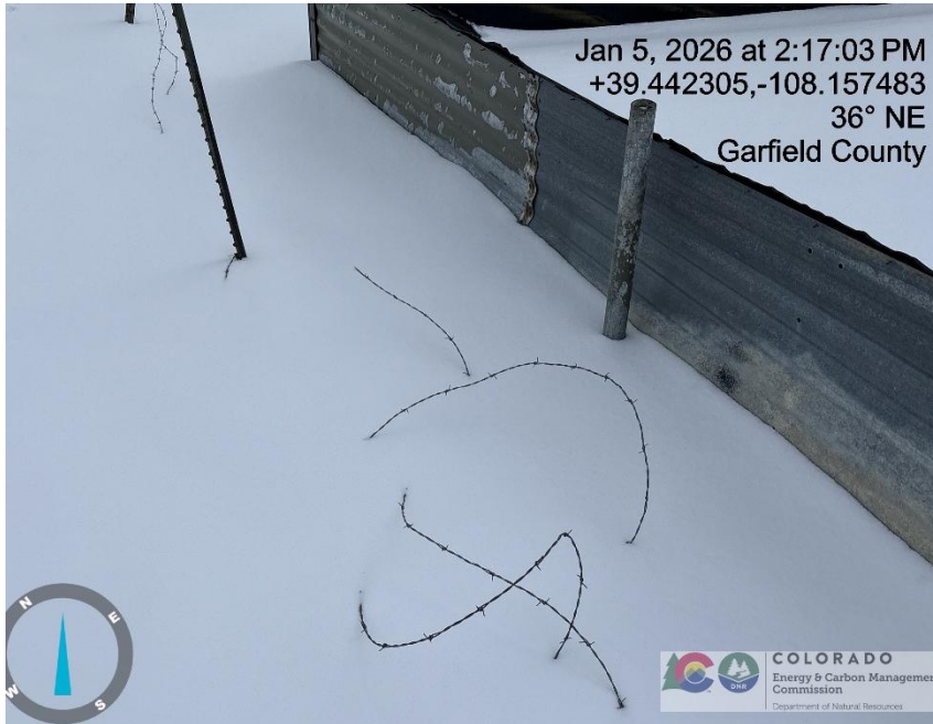
Photo # 8110 Barbed wire fence needs maintenance/wildlife hazard
