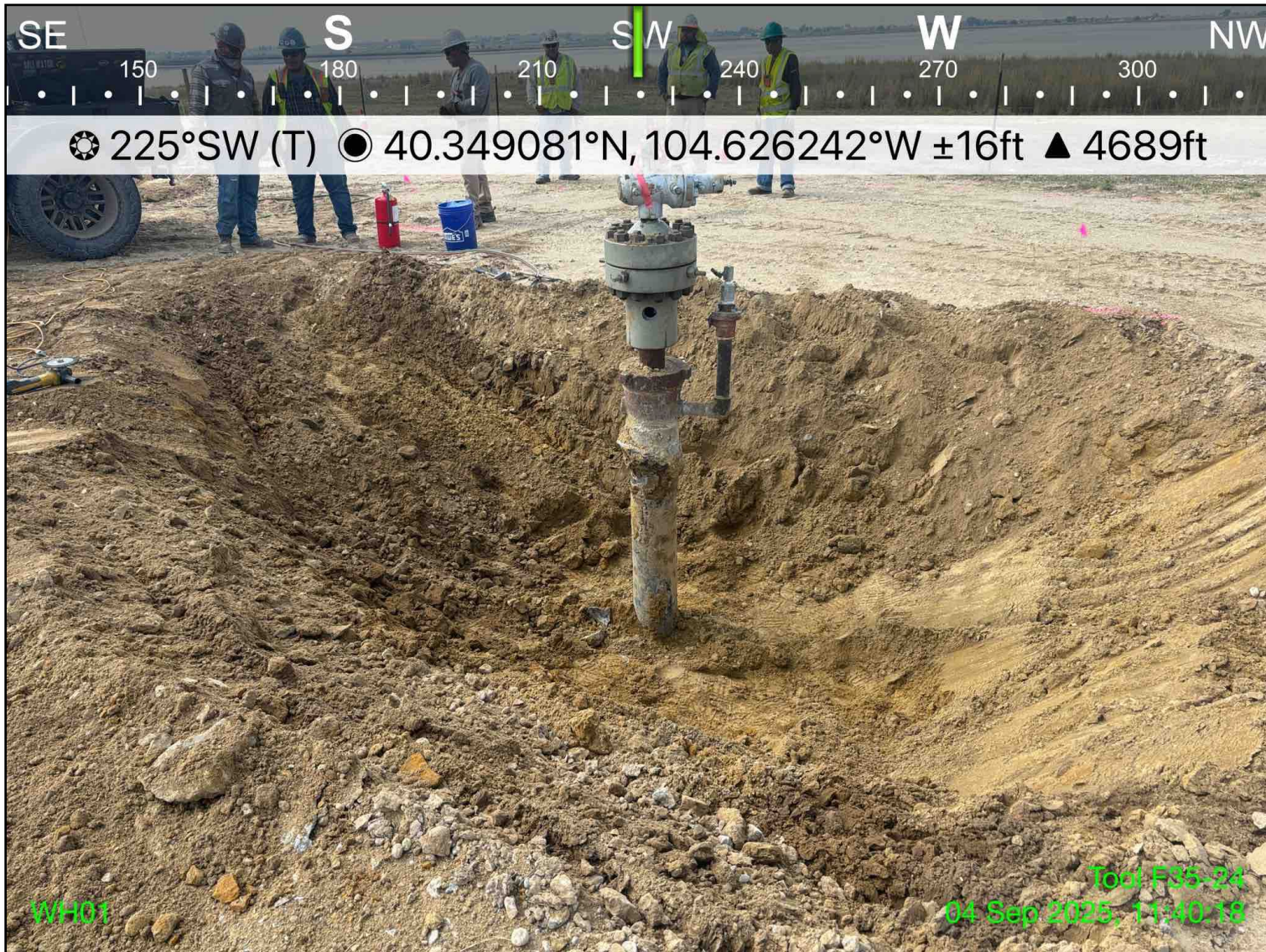
Photo 2: View of wellhead excavation extent, facing southwest
