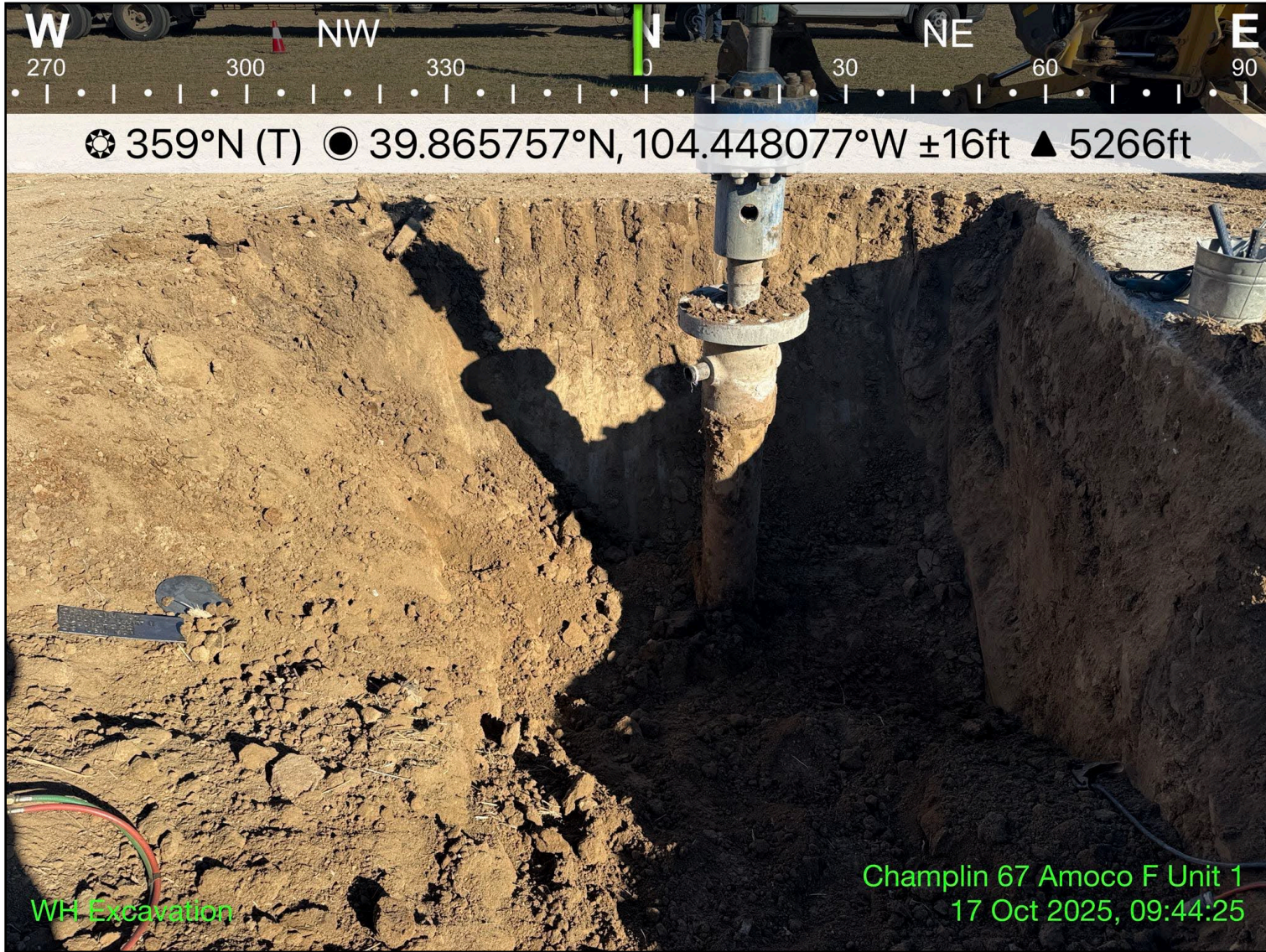
Photo 2: View of wellhead excavation extent, facing north
