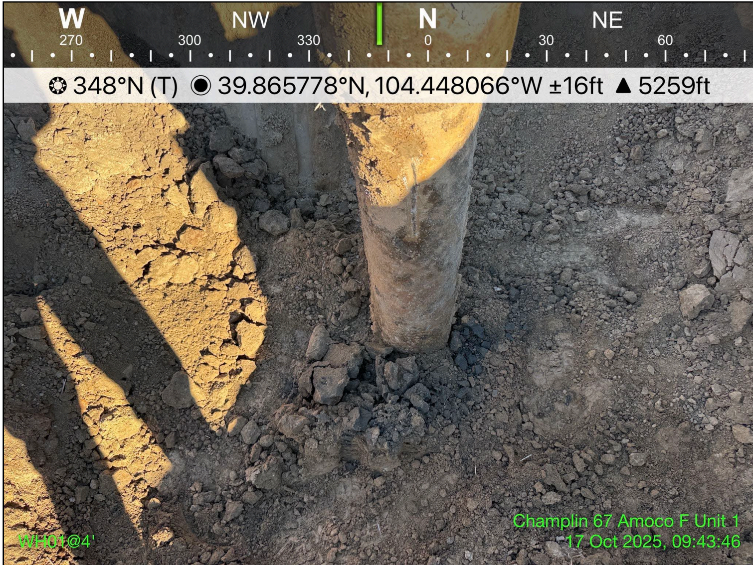
Photo 1: View of wellhead excavation, facing north
