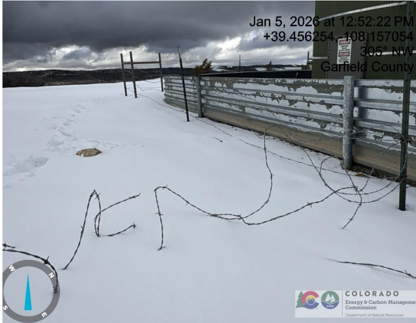
Photo # 7872 Barbed wire fence needs maintenance/wildlife hazard
