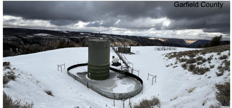
South East corner of location.
